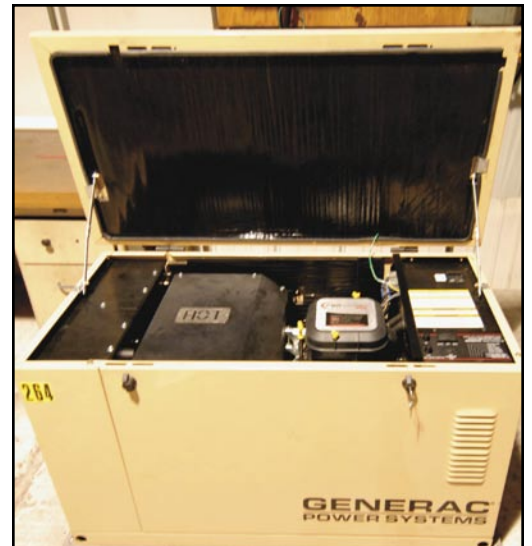
GENERAC 1500 watt natural gas backup generator
