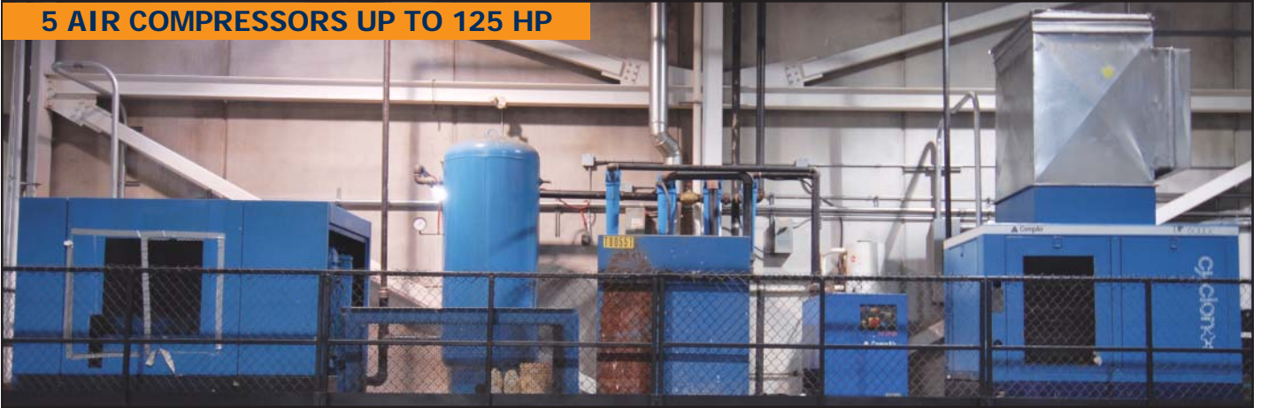
Partial view of air compressors and dryers
