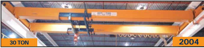
30 TON 2004 MUNCK 30 ton double girder top running bridge crane
