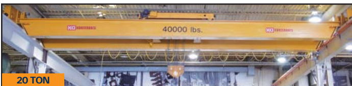
20 TON KONE 20 ton double girder top running bridge crane
