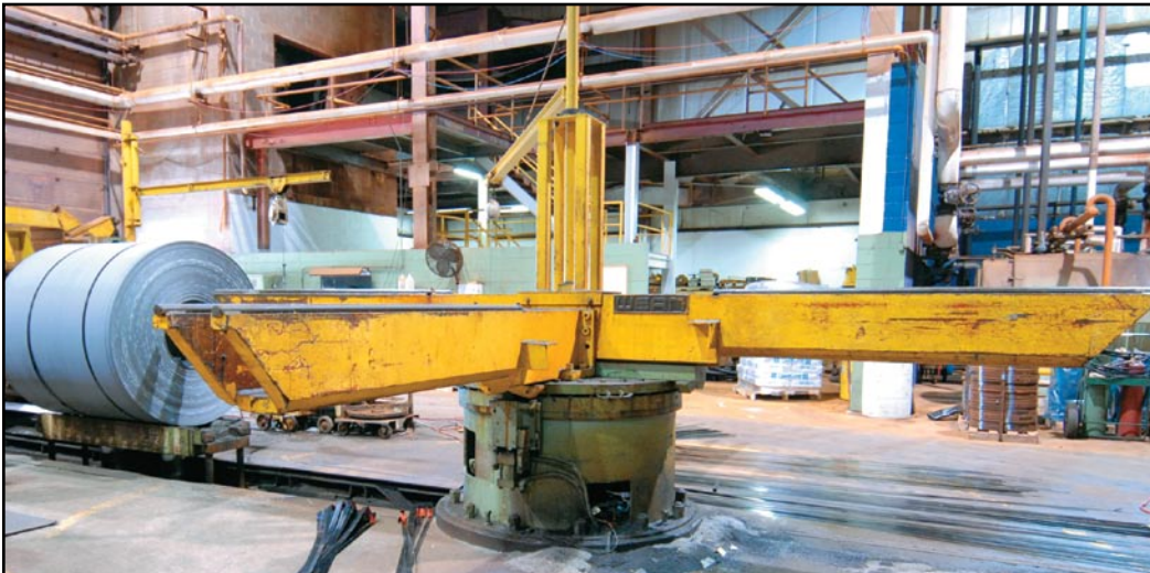
Pit mounted exit coil car, 4 arm turnstile
