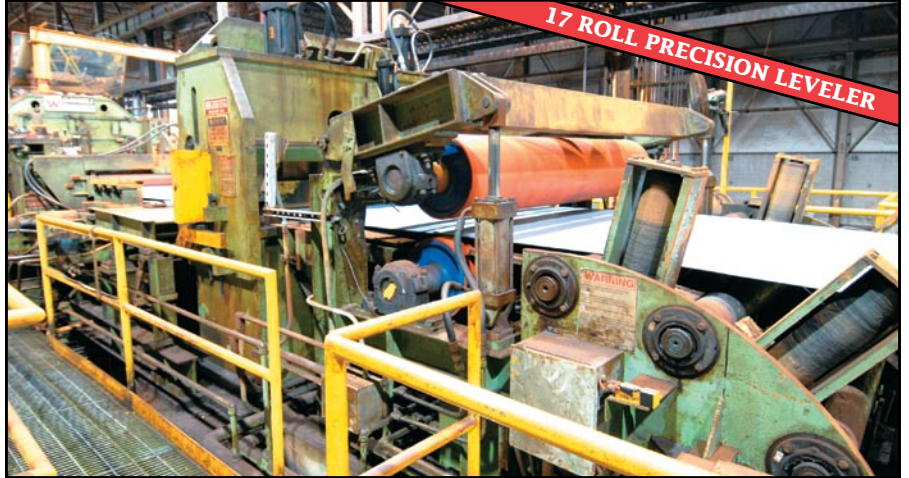
Side guides, pinch roll, steel belt conveyor, 17 roll precision leveler, inspection table, exit parting shear
