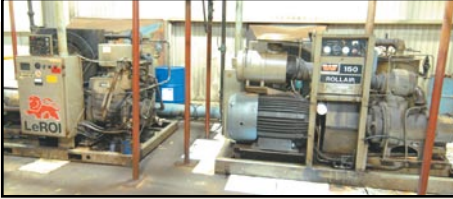
LEROI & WORTHINGTON 150 HP rotary screw water cooled air compressors s/n 4200X93
