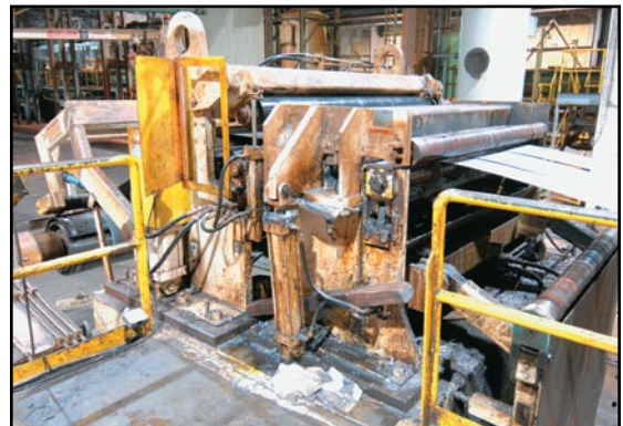
Looping pit table, dual drag pad tension stand, pinch rolls, exit parting shear, exit deflector roll, thread table
