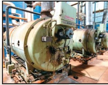
CLEAVER BROOKS gas fired boilers
