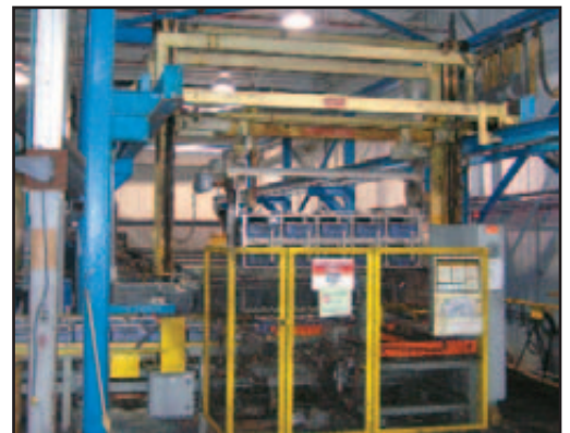
CEF Bright Dip Line & Water Treatment System
